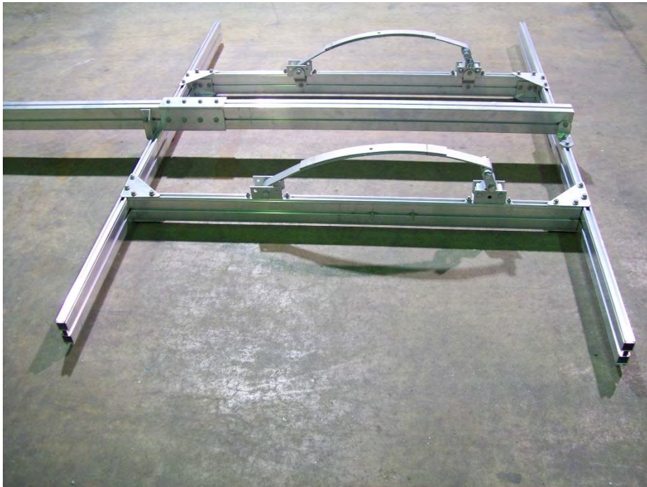
The springs should look like this when properly installed. Do not tighten nuts yet.
